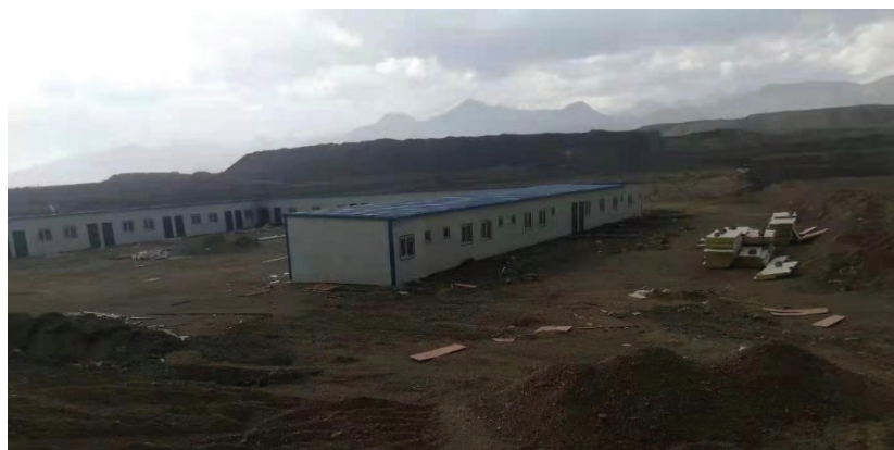
Newly-built staff quarters
